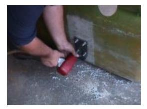
Flat washers and locking washer are used to secure the bracket.
